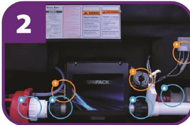
Ensure all plumbing and electrical connections are securely connected and tightened as they can come loose during transit.
