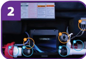
2 Ensure all plumbing and electrical connections are securely connected and tightened as they can come loose during transit.
